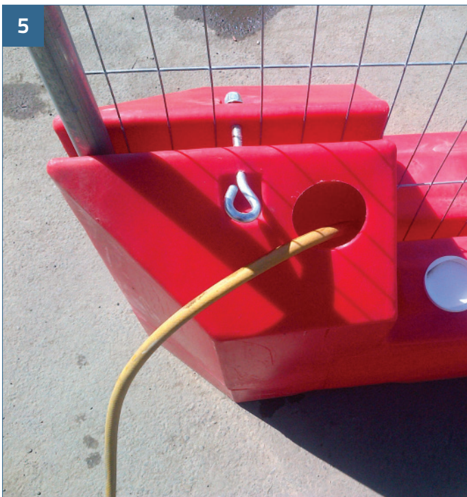
Remove white caps and fill both barriers with water (ensure all white caps are replaced when full).
