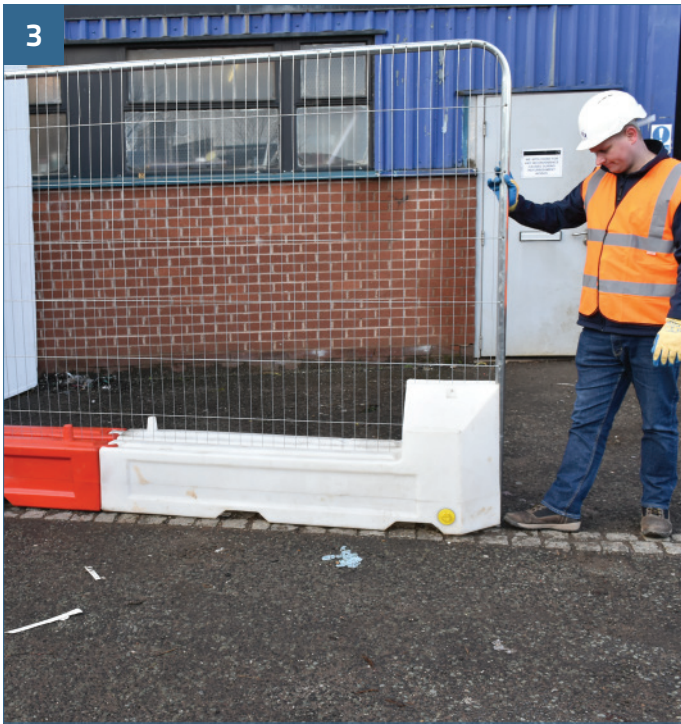
Remove nut and bolt and insert the mesh panel as shown.
