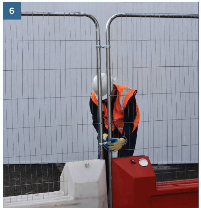
Repeat steps 1 to 5 along your intended installation line, connecting panels with couplers as shown and tighten (13NM).
