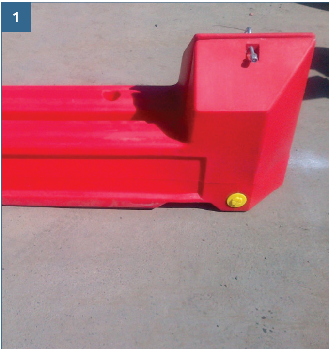
Place first barrier at starting point of intended line of installation.
