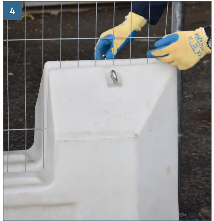
Replace nut and bolt and tighten to secure mesh panel (13NM).
